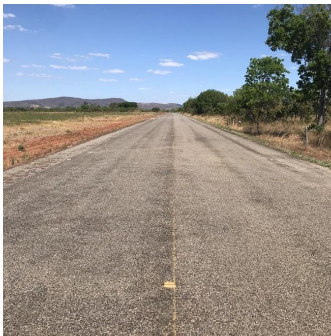
Figura 3 – TO-255, Km 15, Trecho de Porto Nacional a Monte do Carmo – TO.
