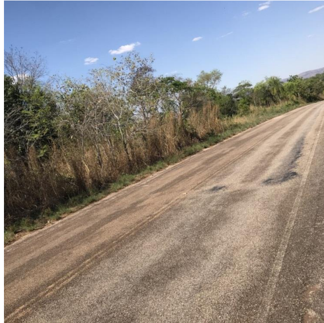
Figura 2 – TO-255, Km 25, Trecho de Porto Nacional a Monte do Carmo – TO.
