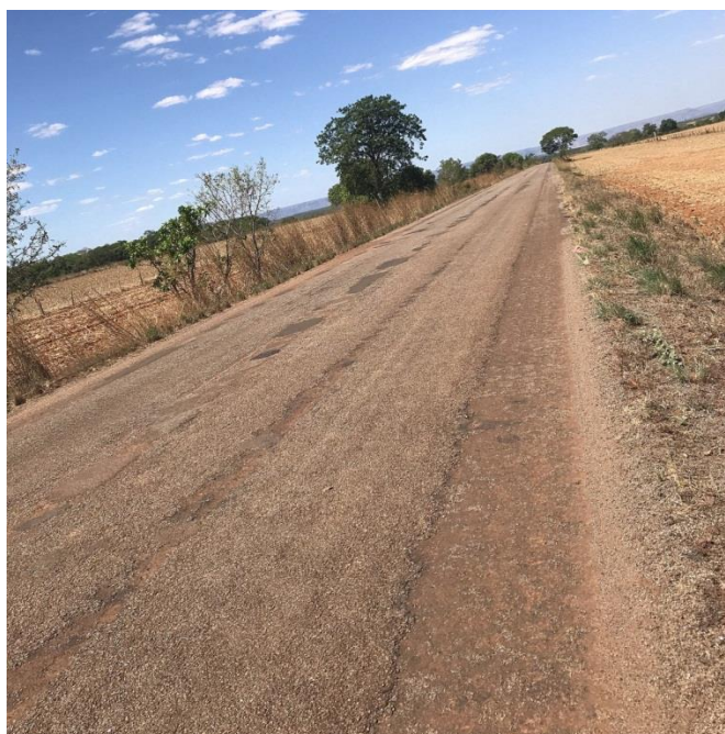
Figura 4 – TO-255, Km 10, Trecho de Porto Nacional a Monte do Carmo – TO.
